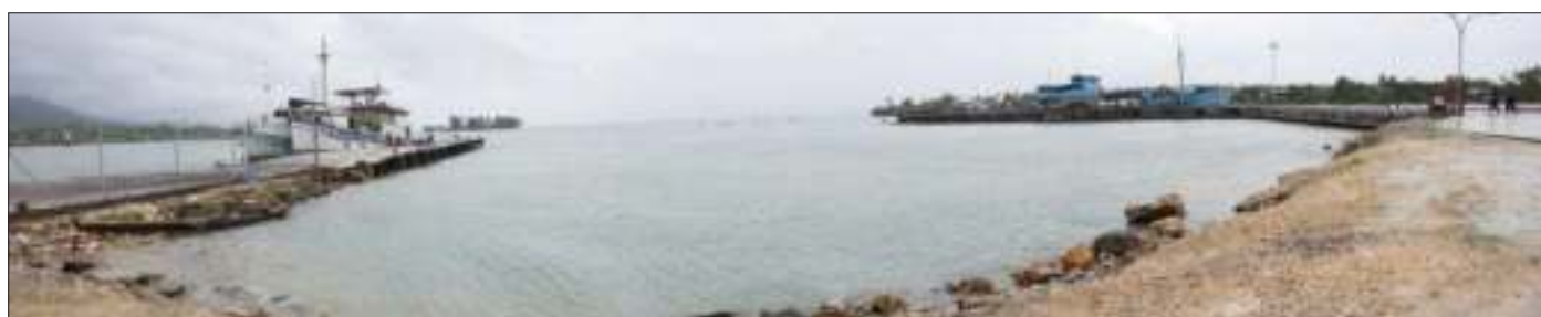
Auki main wharf, Malaita Province
