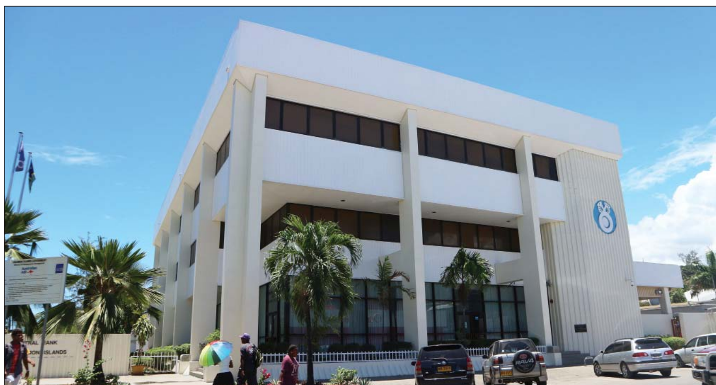
Central Bank of Solomon Islands main Head Office, Mudd Alley street, Point Cruz
